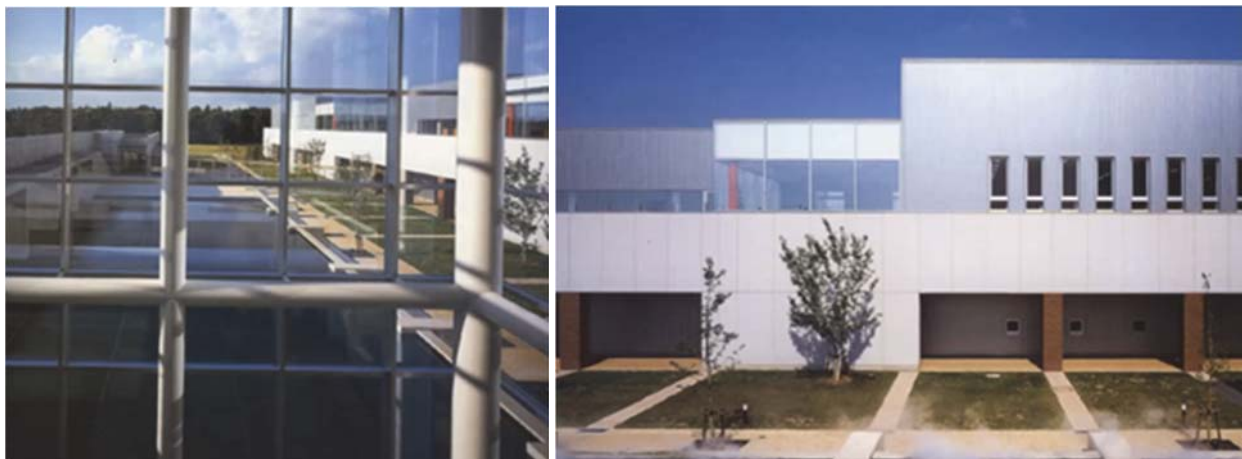
[малюнок. 24-25]. Kurita Water Industries Business & Technology Development Center Tochigi, Japan – Shimizu Corporation (General view, green promenade). [2]
