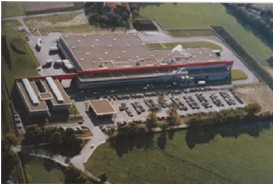
[малюнок.16.] Heinrich Nolke GmbH & Co Meat Processing Plant Versmold, Germany ATP Achammer – Tritthart & Partner, architects and engineers. [2]
