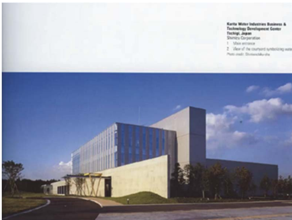
[малюн.22]. Kurita Water Industries Business & Technology Development Center Tochigi, Japan – Shimizu Corporation. [2]
